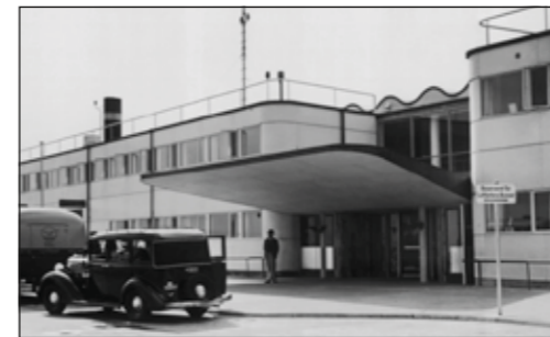
Overhang entrance Kastrup Airport Terminal
